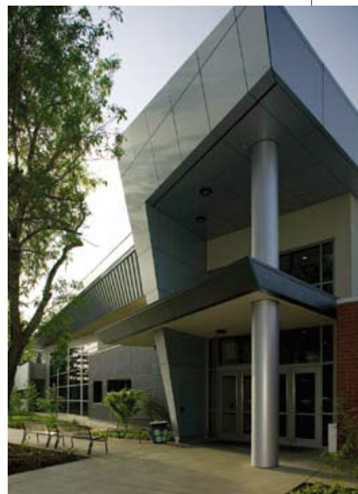
This $8.4 million dollar project was a winner of one of the WCCC's 2007 Distinguished Project Awards. It is the American River College Learning Resource Centre, located in Sacramento, CA., and was completed in 2005. Photo by Todd Quam, Digital Sky Aerial Imaging.
