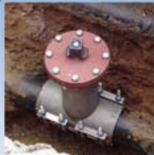
Permanent Valve Insertion with Insta-Valve Plus
