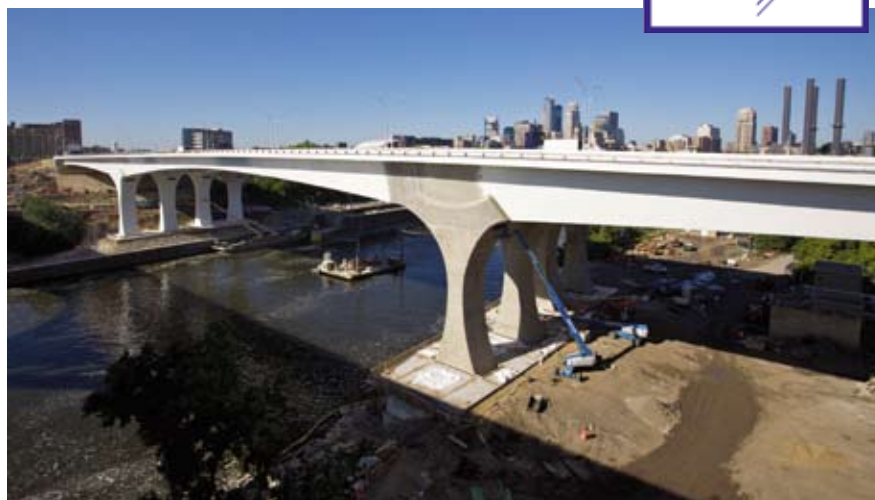
The new I-35W Mississippi River bridge officially opened September 2008. DBIA member James McHugh Construction Co. was the design-builder and constructor on the project. DBIA member Wight & Co. was the engineer.
